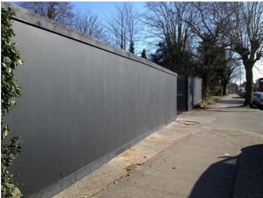
Figure 6: Example of Suitable Hoarding
