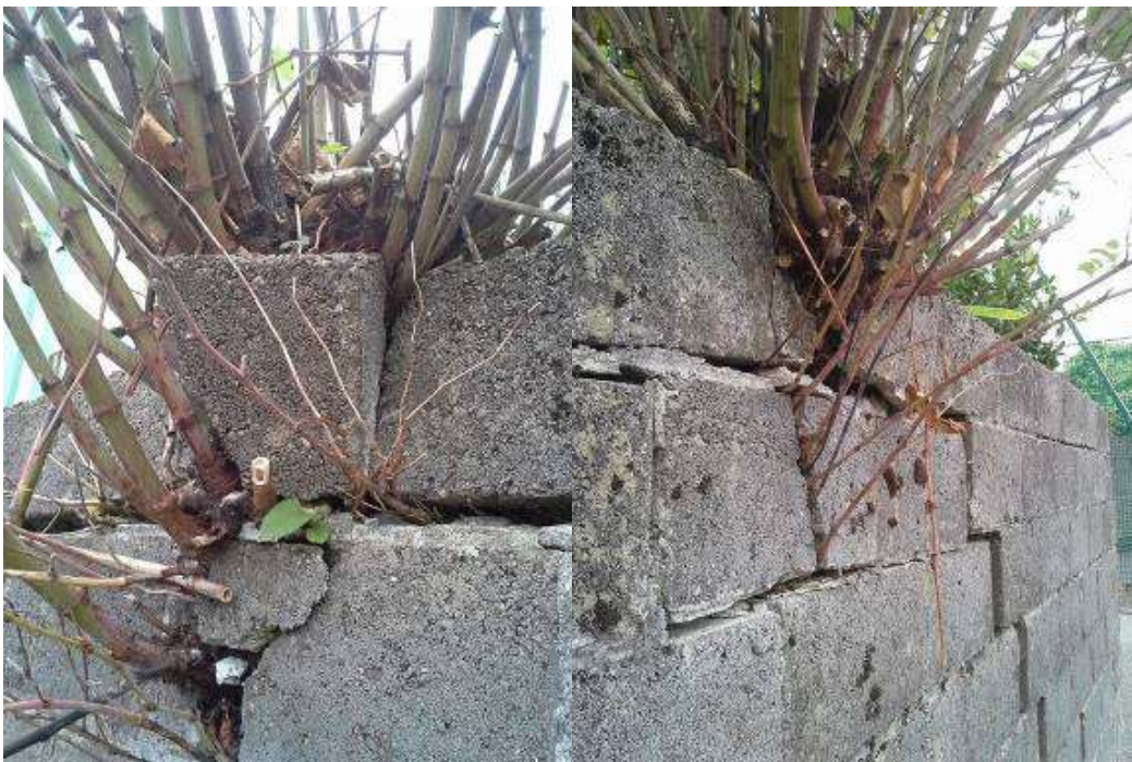
Photograph A.4 Japanese Knotweed breaking through cavity blocks resulting in a structural crack in the wall of a garden in Co. Cork (Source: Lisa M. J. Dolan, Ecosystem Services)
